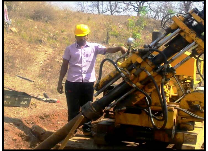
Commencement of drilling
