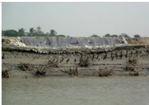
Severe erosion showing exposed mudflats. Bakkhali sea beach
