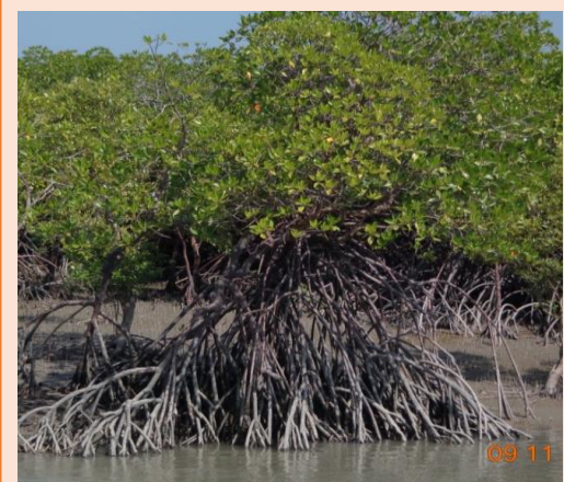
Exposed mangrove roots showing severe erosion – a threat to the landmass and a common feature of Sundarbans.
