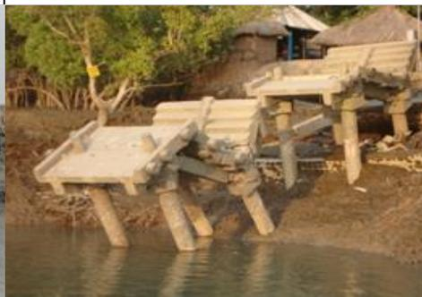
Collapse of concrete jetty due to bank failure in Vidya river
