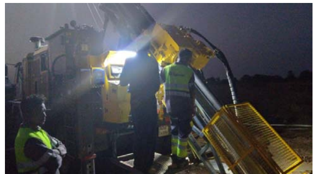
Drilling operation in progress.
