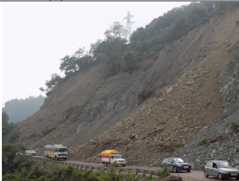
Field Photograph of Dattyar Village Slide at RD of 71+100 to 71+200 along NH-22
