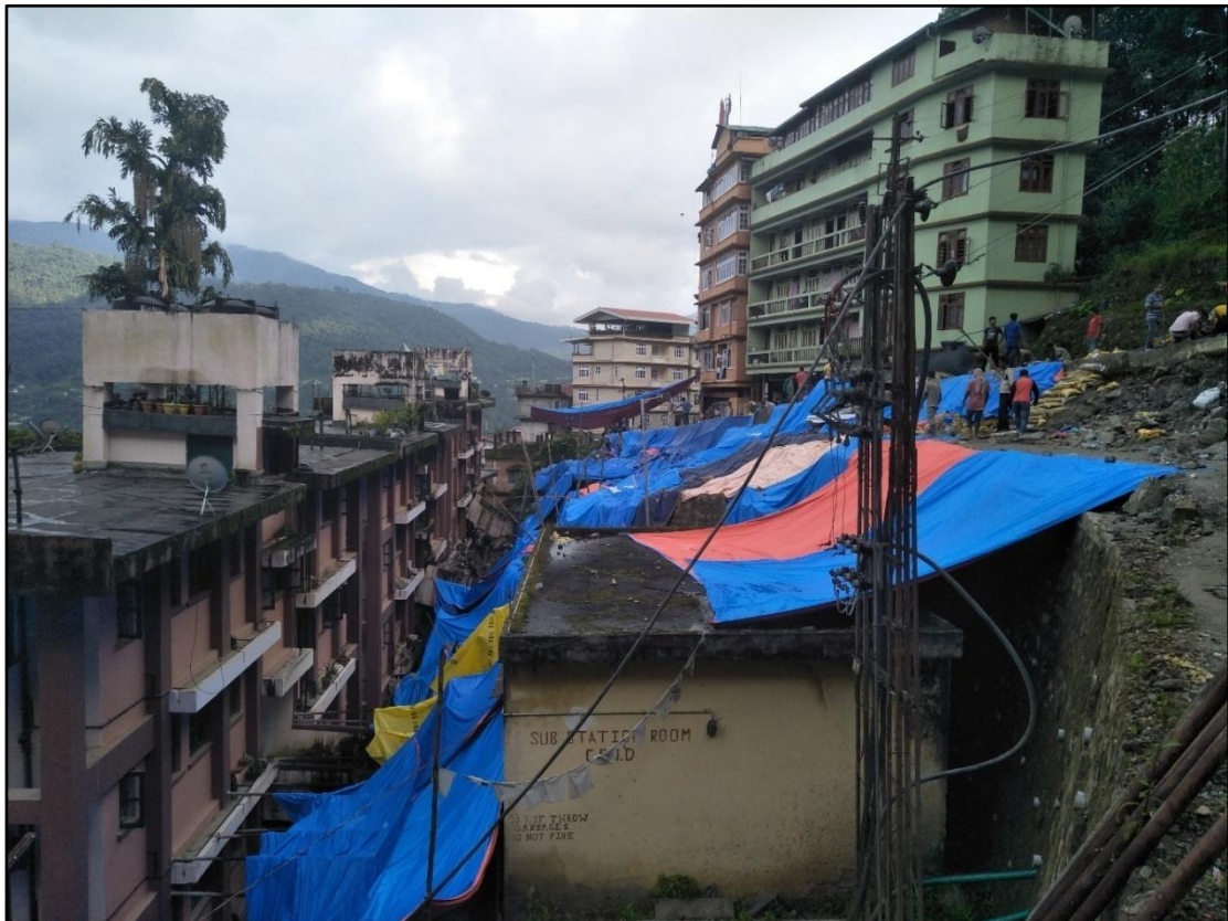
Fig 2: The affected slope due to failure in Upper Syari.
