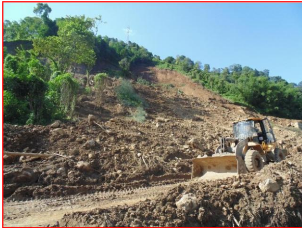
Fig-1: Laptap Landslide, PapumPare District, Arunachal Pradesh
